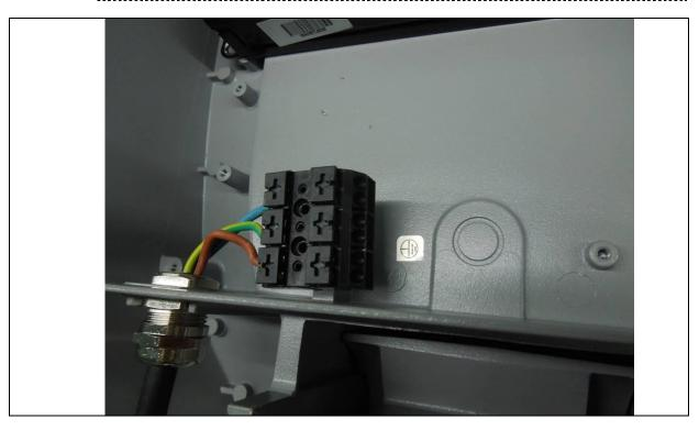
Details of: Earthing terminal internal view
